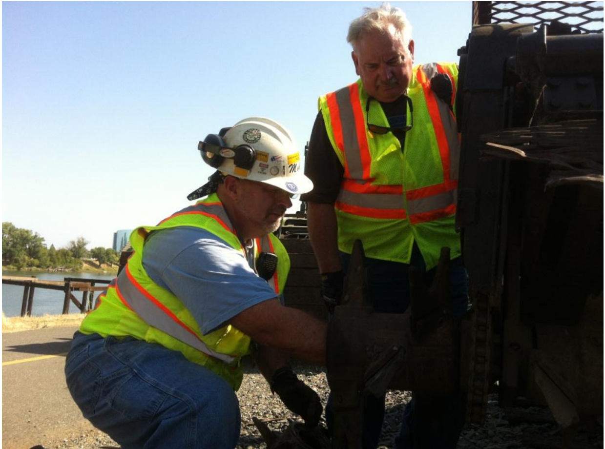
Mike F. and Harry install an extension drum on the scarifer
