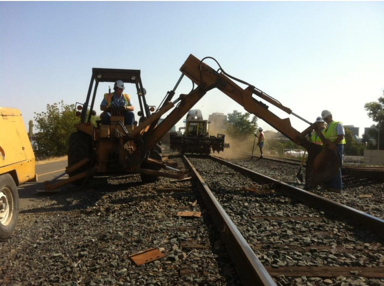
MOW machine team at work: back-hoe and scarifer working in tandem
