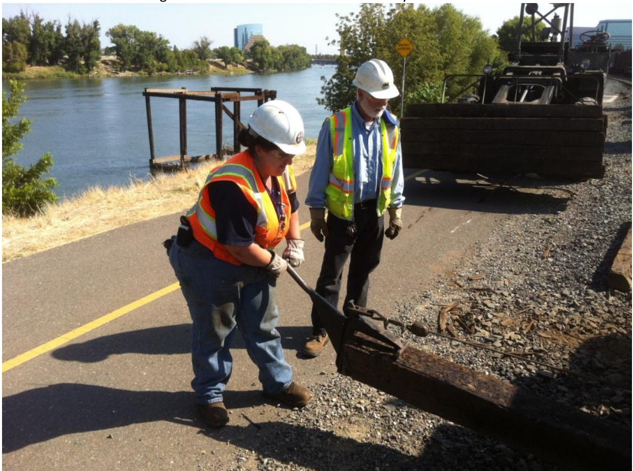
Heather and Mike M. use the inserter function of the scarifer to insert a new tie
