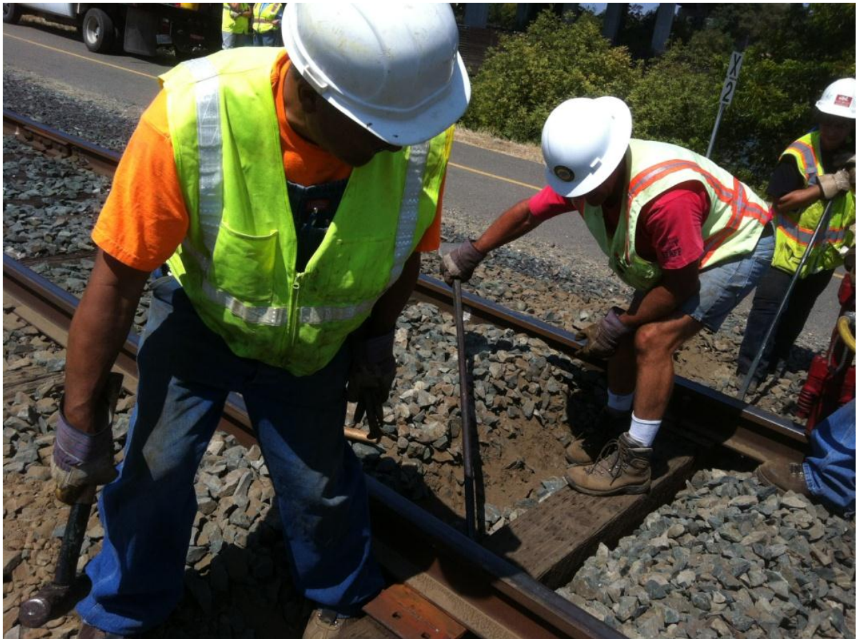
John Rexroth and Steve Mathais “nip” the rail to insert a tie-plate
